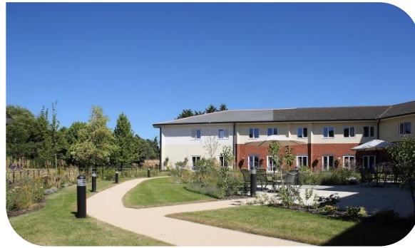
2. SHINFIELD VIEW (READING)
