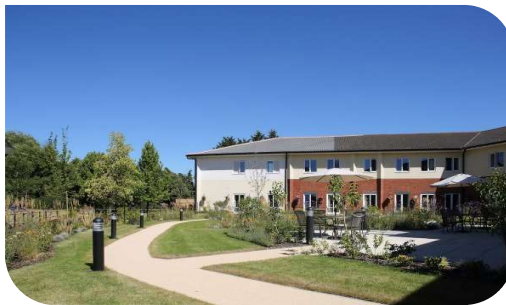
2. SHINFIELD VIEW (READING)
