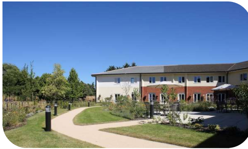
2. SHINFIELD VIEW (READING)
